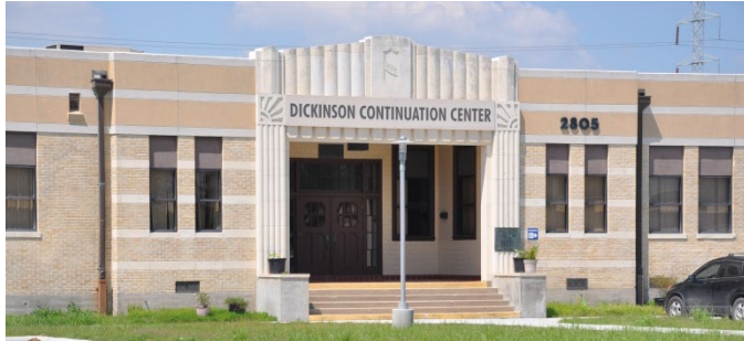
Renovation of a historic building for DCC and DALC
