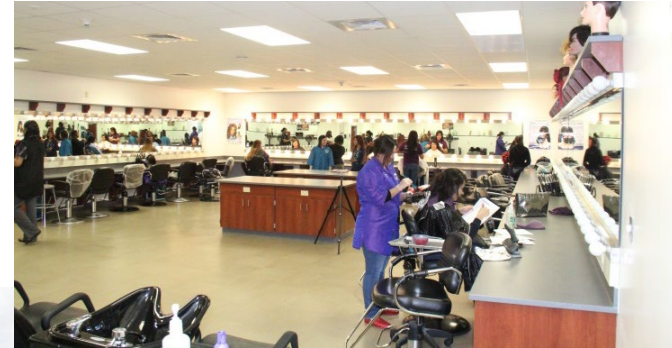
A portion of the Career and Technology wing renovation
